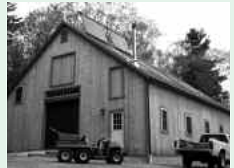
Solar hot water panels on the Maintenance Building.
